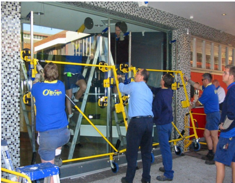
Using 2 Nomads to install a heavy plate of glass
